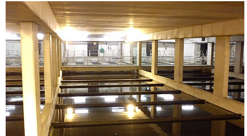
Anammox technology in low temperature wastewater at WWTP Holland
